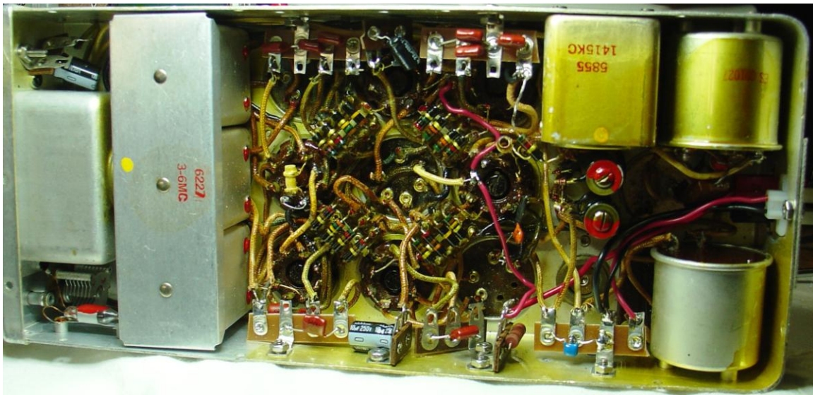
Figure 3: Bottom view of the re-wired and re-capped receiver
