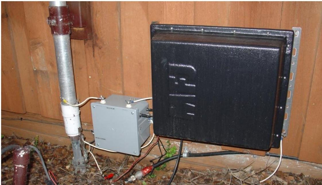
Figure 7: MFJ-998RT and remote-switched inductor extender at base of 43-foot vertical
