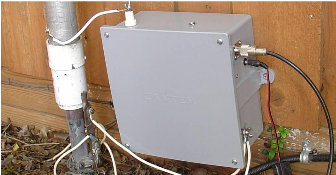
Figure 17: 160/80M matching unit feeding the author's 43-foot vertical
