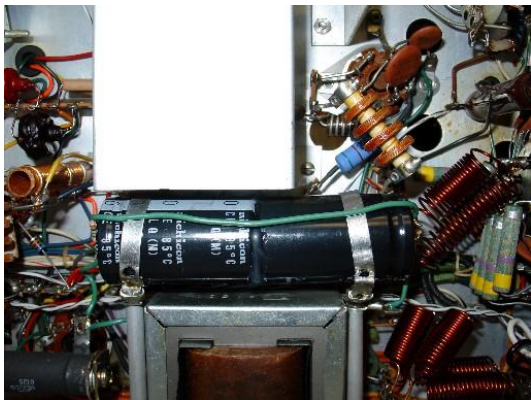
HV Capacitor and Grid Resistor
