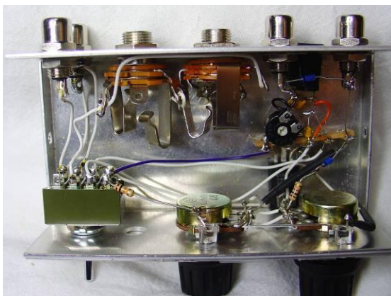
Figure 3: Interior view of the unit
